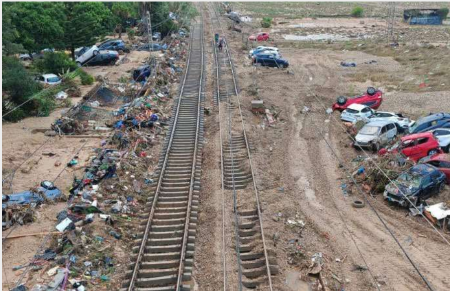
Figure 13: Flood in Valencia, ADIF, 2024
