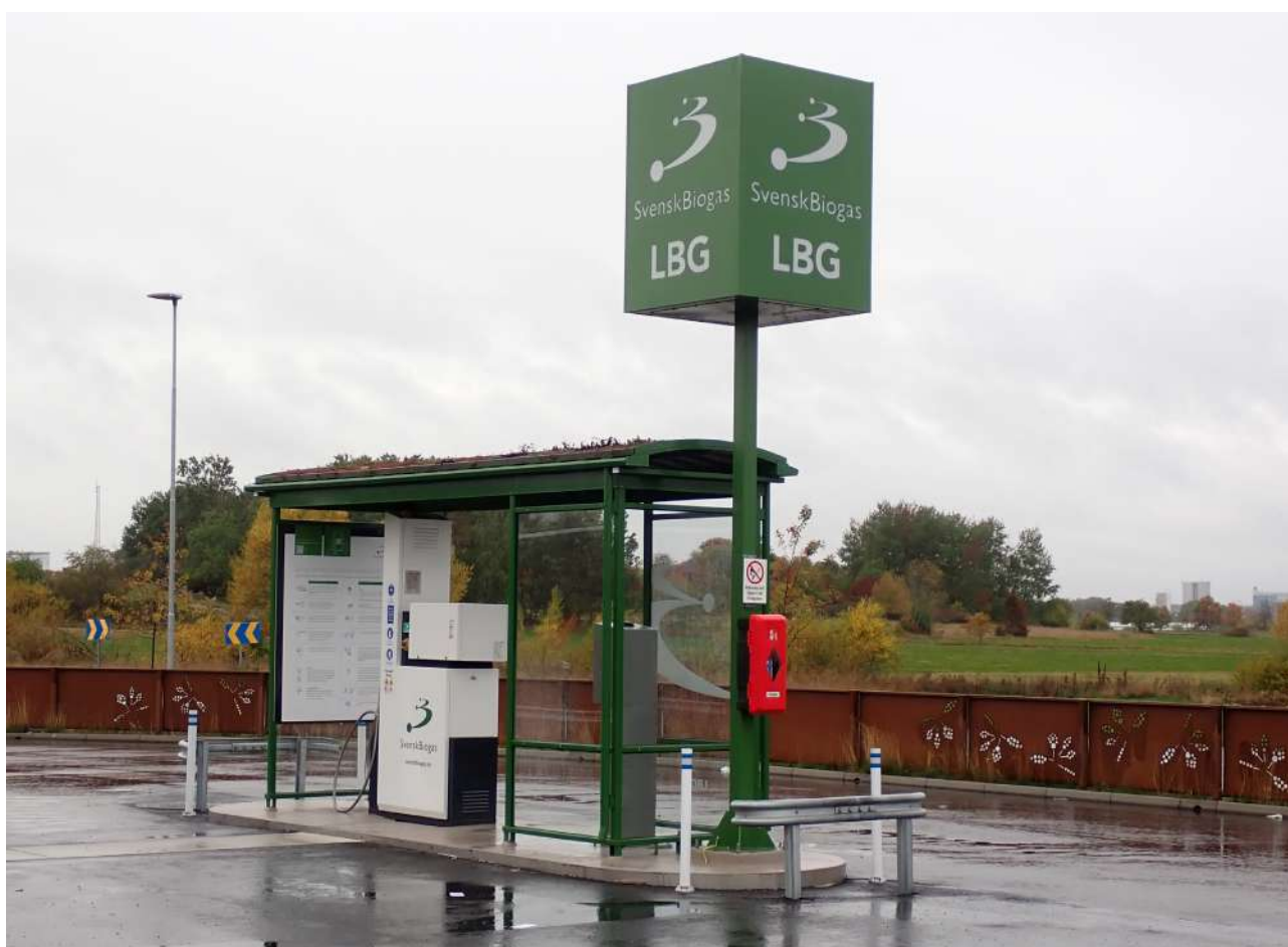
Figure 7. LBG Station in Linköping. © Peter Kornatz
