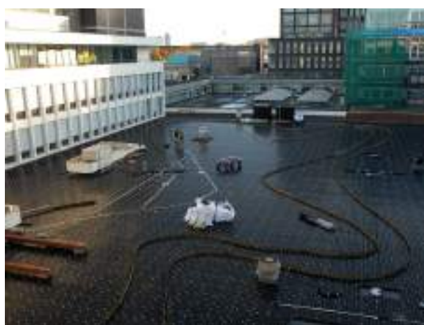
A smart blue-green roof under construction (left) and finalised (right) © Dakdokters
