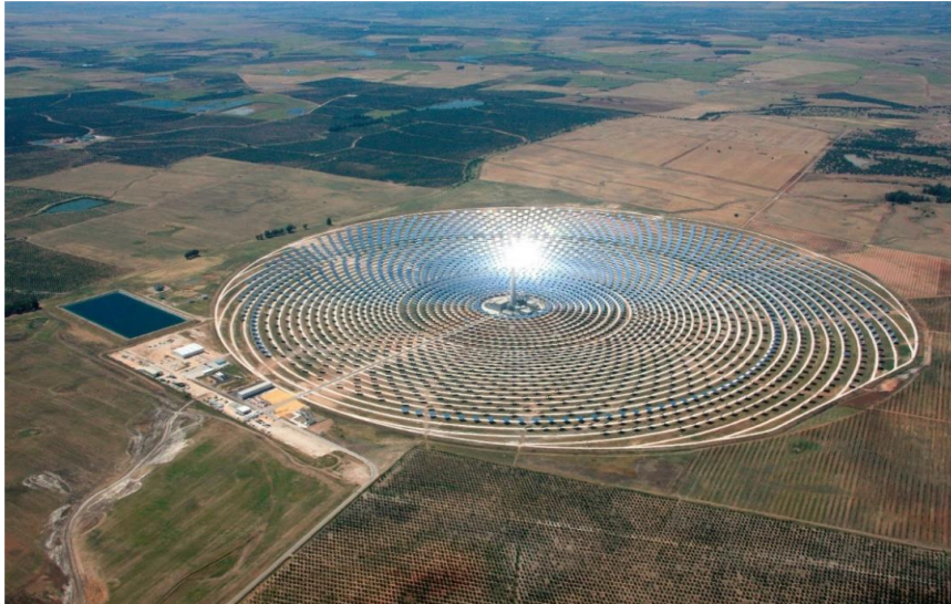
Figure 10: Aerial view of Gemasolar plant.
