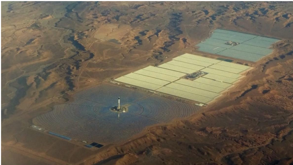
Figure 6: Aerial view of the Noor complex
