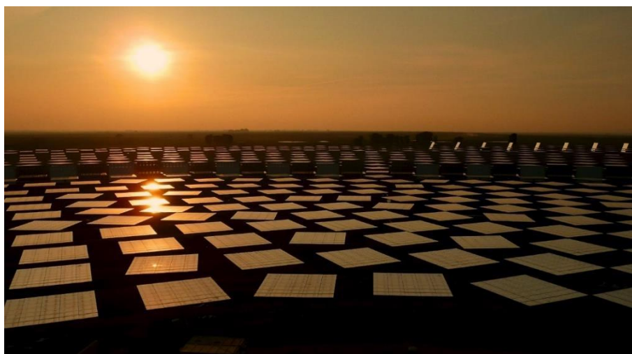
Figure 12: View of the heliostat field with the first rings in "defense" (flat) position.
